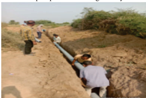
g. Installation of underground pipeline in farmers field
