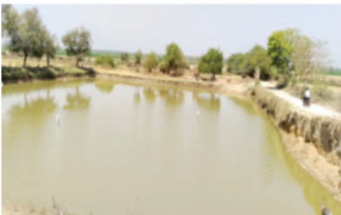
a. De-silted water harvesting structure in the watershed
