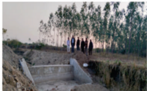
b. Repair of inlet and outlets of the water harvesting structure
