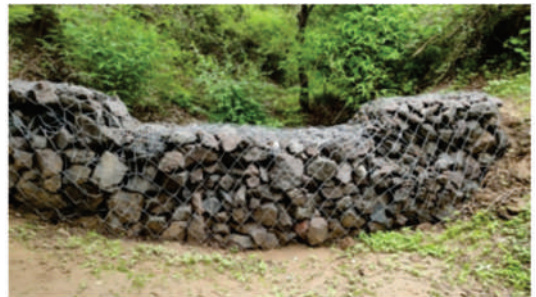
Gabion structure + bamboo
