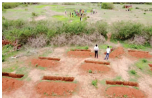
Staggered trenching
