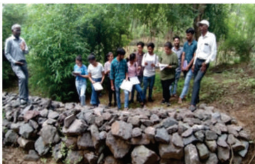
Loose boulder check dam
