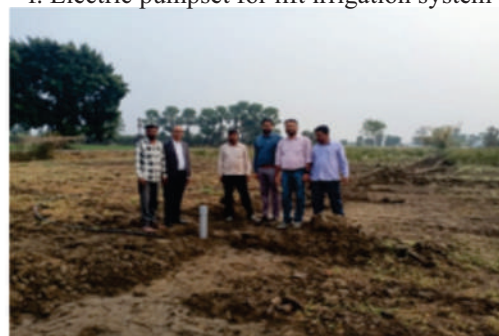
h. Outlets of underground pipeline in farmers field
