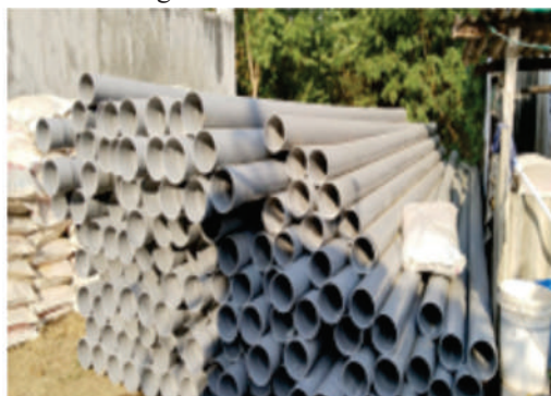
d. PVC pipes for underground pipeline network
